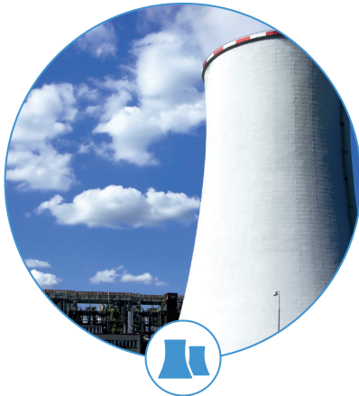
ELECTRICAL POWER GENERATION
