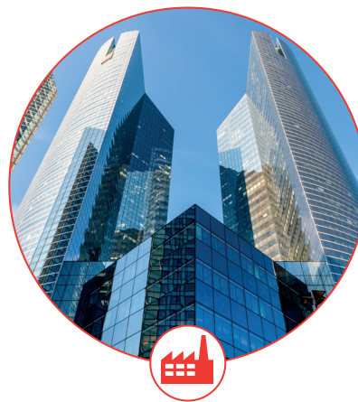
INDUSTRY AND TERTIARY BUILDINGS
