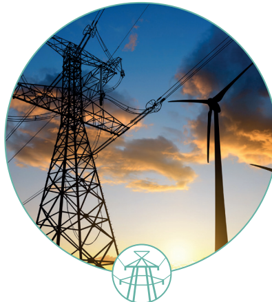
ELECTRICAL POWER TRANSMISSION AND DISTRIBUTION
