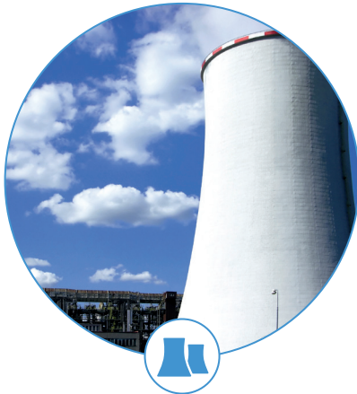
ELECTRICAL POWER GENERATION
