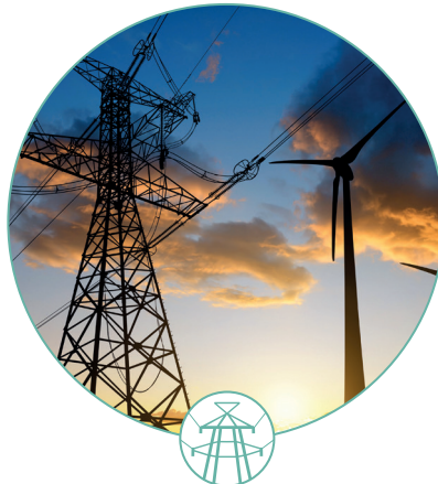
ELECTRICAL POWER TRANSMISSION AND DISTRIBUTION
