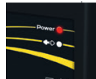
COM LED: data exchange on the RS485 (flashing according to RS485 transmission speed)
